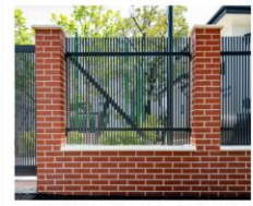
#3: LOW BRICK WALL WITH FENCE ABOVE
