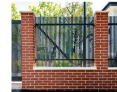
#3: LOW BRICK WALL WITH FENCE ABOVE
