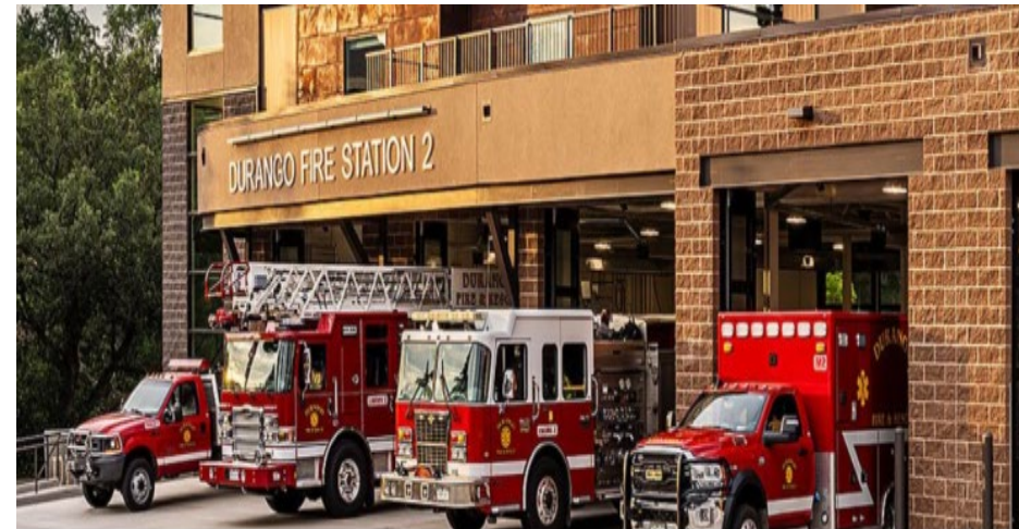
FCI – Durango Fire Station No. 2
