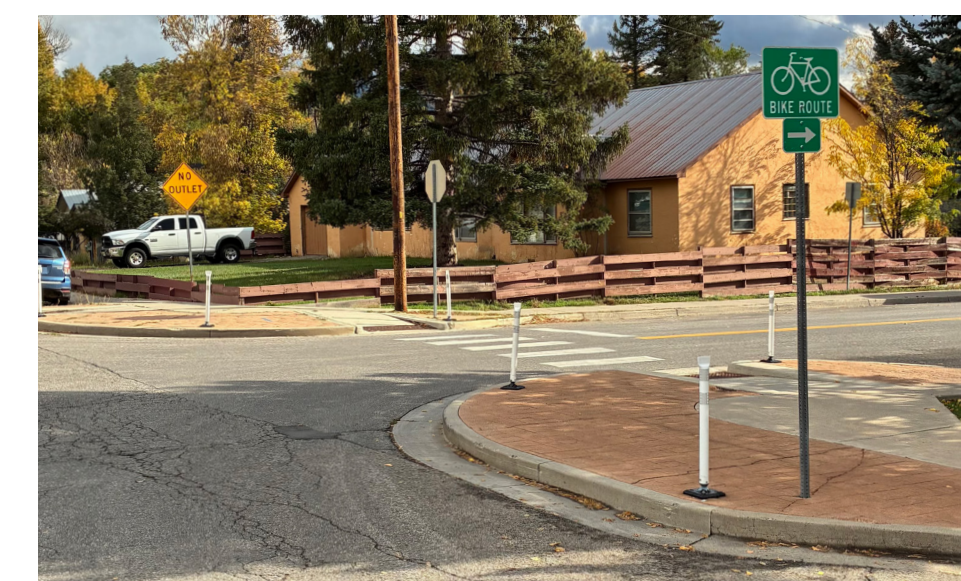
Curb extensions near Needham Elementary on West 24th St. and West 3rd Ave.
