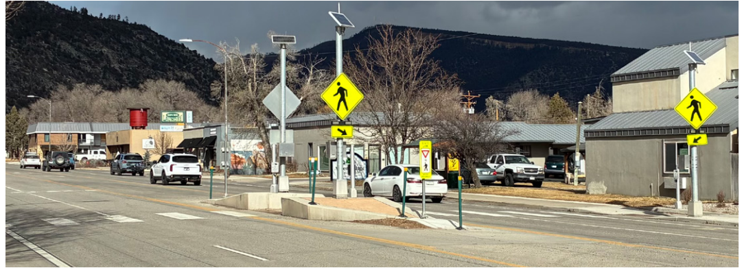
Photo 37. Median with pedestrian refuge on Camino Del Rio at W 7th Pl, Durango, CO
