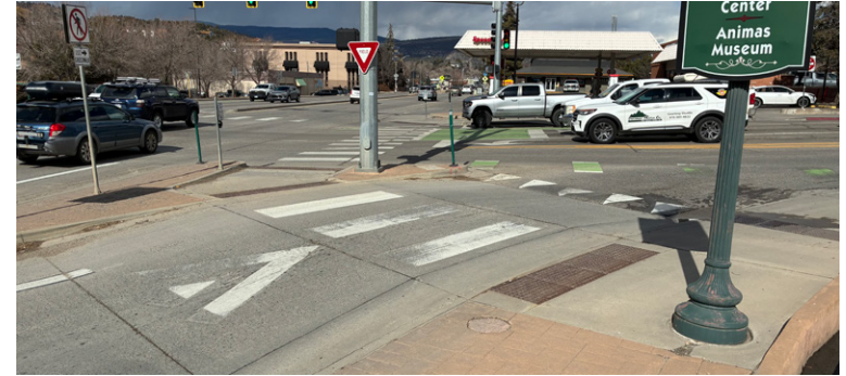
Photo 16. Concrete raised crosswalk at intersection
