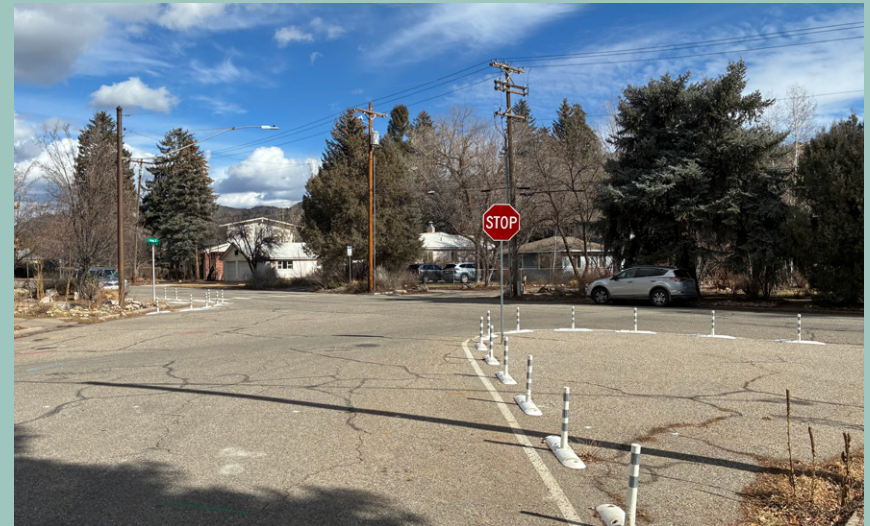
Photo 30. Realigned intersection at W Park Ave and Alamo St
