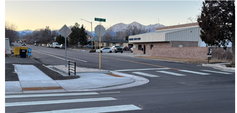
Photo 24. Concrete curb extension
