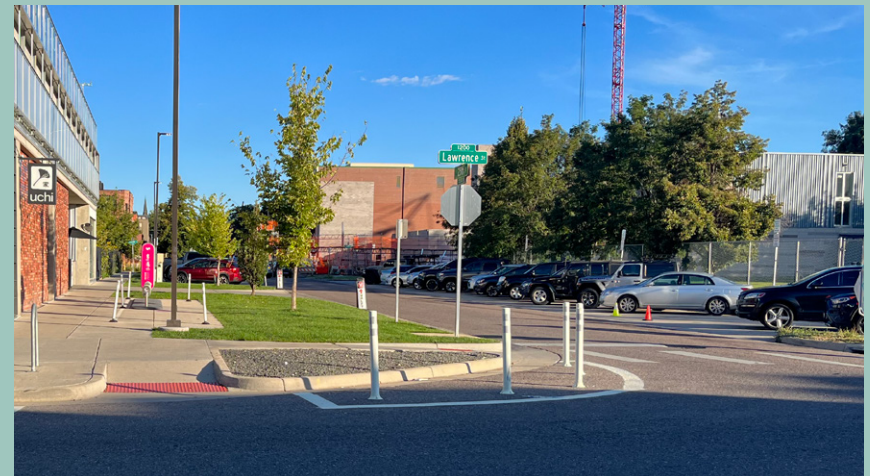
Photo 28. Turn wedge using paint and flexible posts
