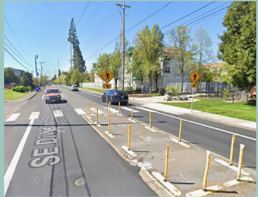
Photo 38. Pilot median island using paint and flexible posts.
