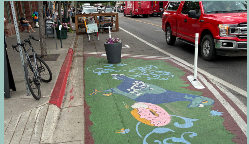
Photo 25. Curb extension using paint and flexible posts.
