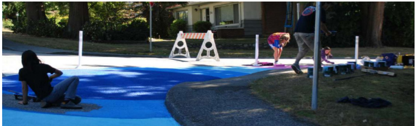
Photo 14. Installation of pilot project.
