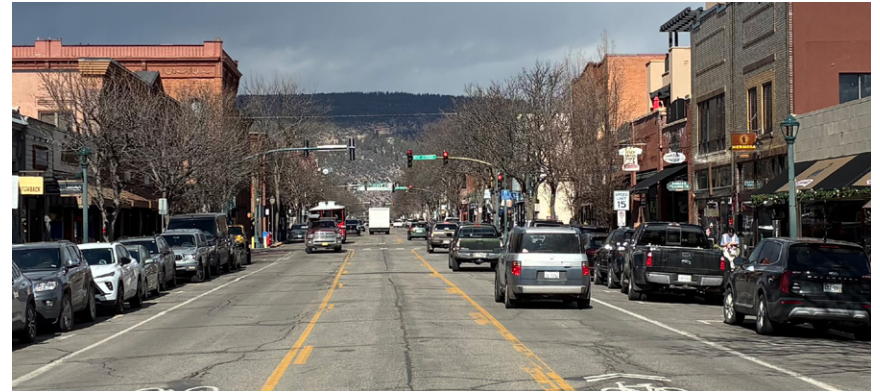
Photo 40. Four- to three-lane conversion on Main St, Durango
