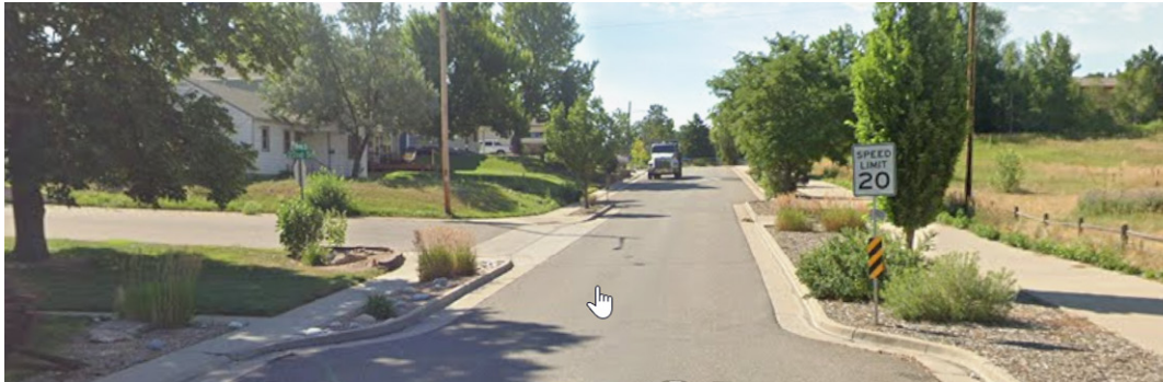
Photo 20. Pinch point at an intersection.
