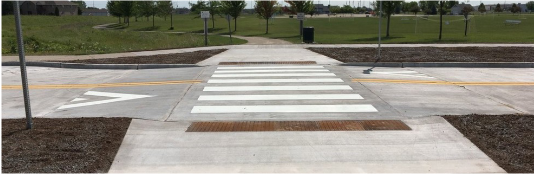
Photo 15. Concrete raised crosswalk at mid-block location
